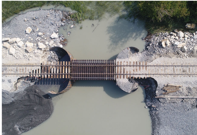
High water scoured bridge infrastructure, including at MP 16.2, seen here from the side and above.
