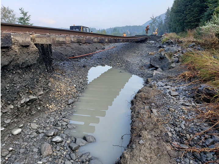
Track maintenance crews tackle several areas impacted by significant washouts from high water.
