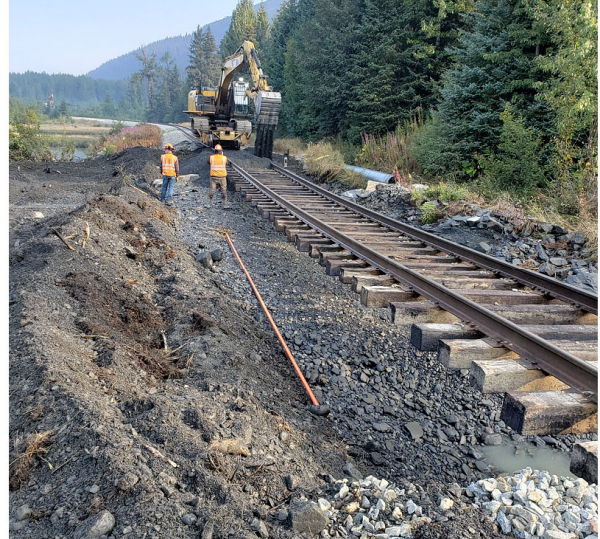
Track maintenance crews tackle several areas impacted by significant washouts from high water.
