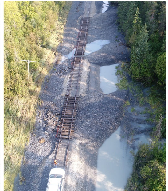
Snow River rising water flows over the tracks. Later over the weekend receding water reveals track washouts.
