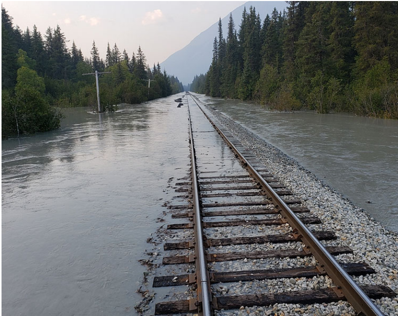
Snow River rising water flows over the tracks. Later over the weekend receding water reveals track washouts.
