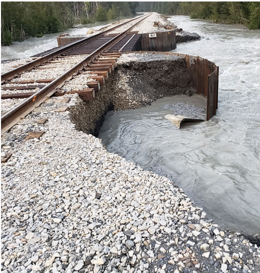
High water scoured bridge infrastructure, including at MP 16.2, seen here from the side and above.
