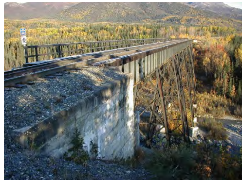
Riley Creek Bridge (photo courtesy of ARRC)
