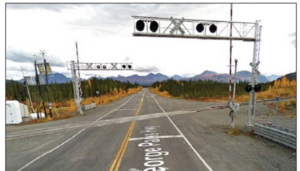
At-grade crossing at ARRC Milepost 345.09.
