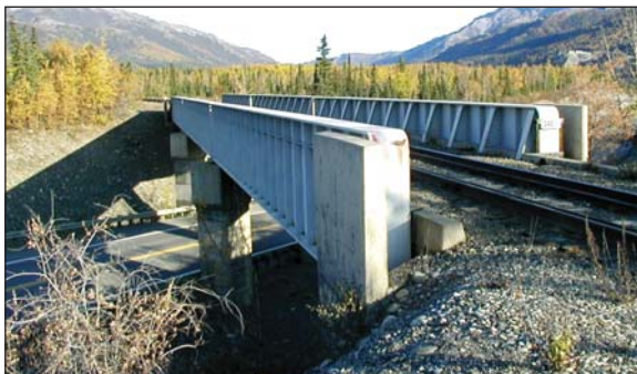
Rail-over-road crossing at ARRC Milepost 346.71.
