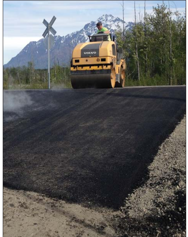
The Matanuska Spur Road crossing is paved after crossing improvements are completed in 2014-2015.
