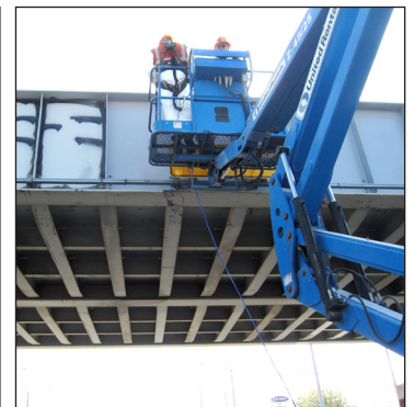
The Dimond Blvd rail bridge is repainted after cleaning in 2011.
