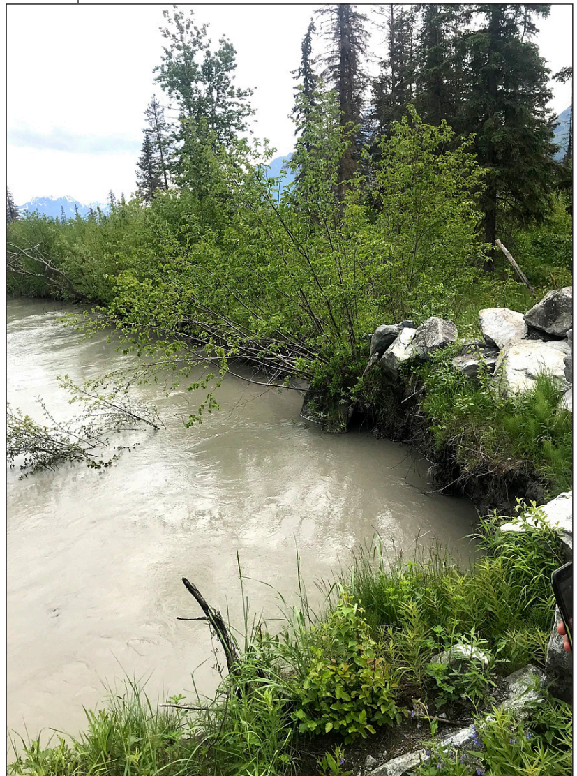
The earthquake damaged and destabilized parts of the track embankment adjacent to the Knik River, which flows under railroad bridge 147.5.
