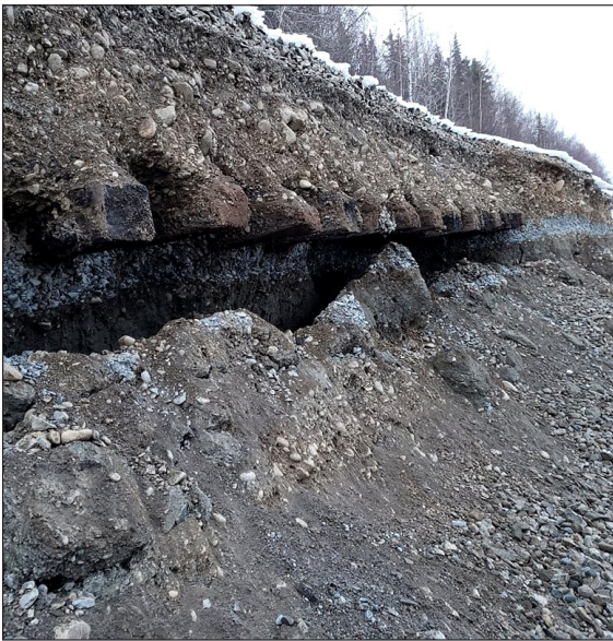
The 2018 earthquake caused extensive shoulder and sub-structure damage to track infrastructure.
