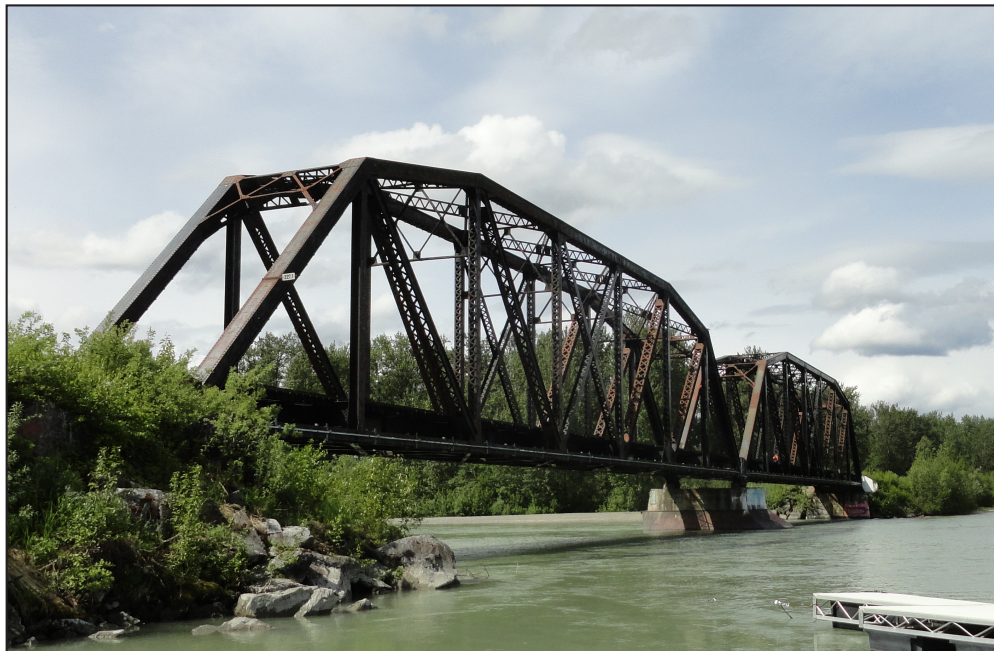
The 406-foot bridge features two steel through-truss spans that will be rehabilitated.
