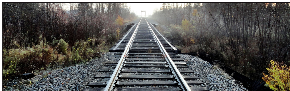
Project work will include full replacement of the existing bridge with three culverts.
