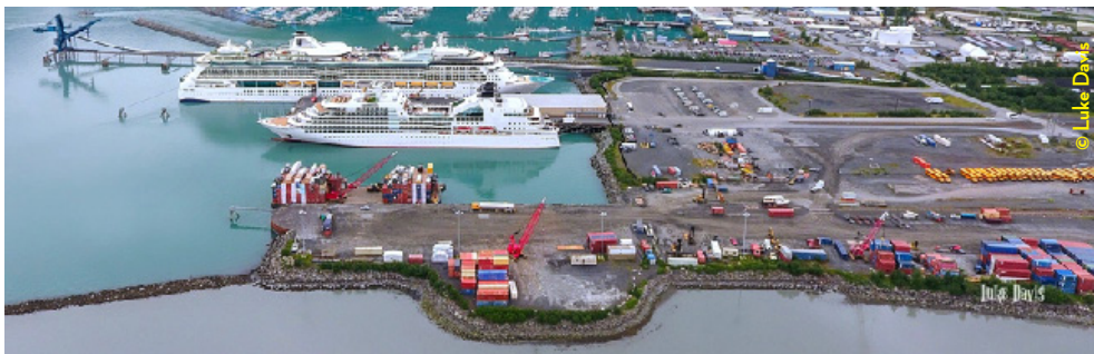
The Freight Dock with Passenger Dock in the background.
