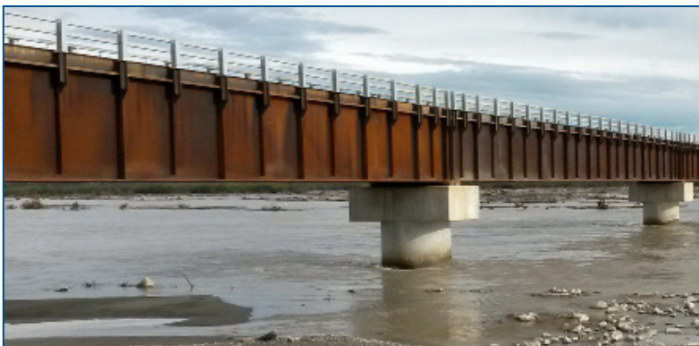
Left: A bridge showing deck plate girder spans, similar to the 175-foot span that will combine with two 65-foot beam approach spans to replace Bridge 351.4. Right: A drawing of a deck plate girder bridge from the American Railway Engineering and MOW Association (AREMA).
