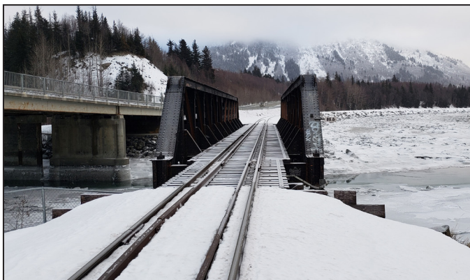
Above: The pony truss and timber trestle bridge at MP 86.6 over Bird Creek will be replaced with a single thru-plate girder span (see drawing at right for reference).
