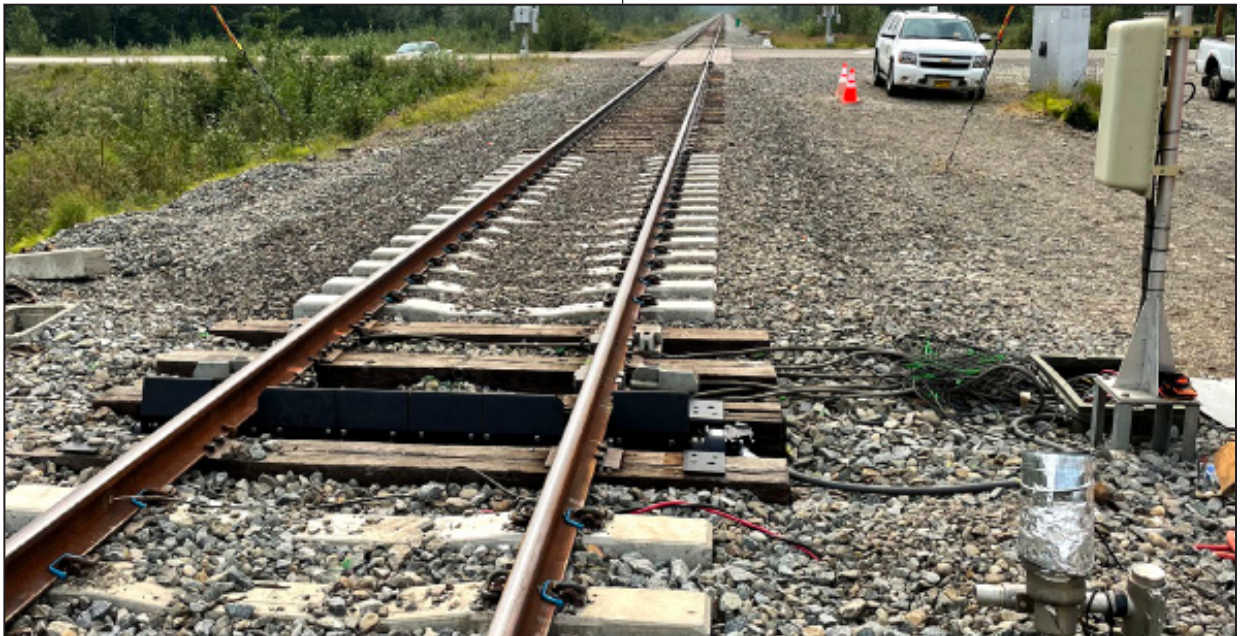
Pictured, an existing detector site along the Alaska Railroad. The 45 sites receiving upgrades with locations can be viewed on the map on page 2.
