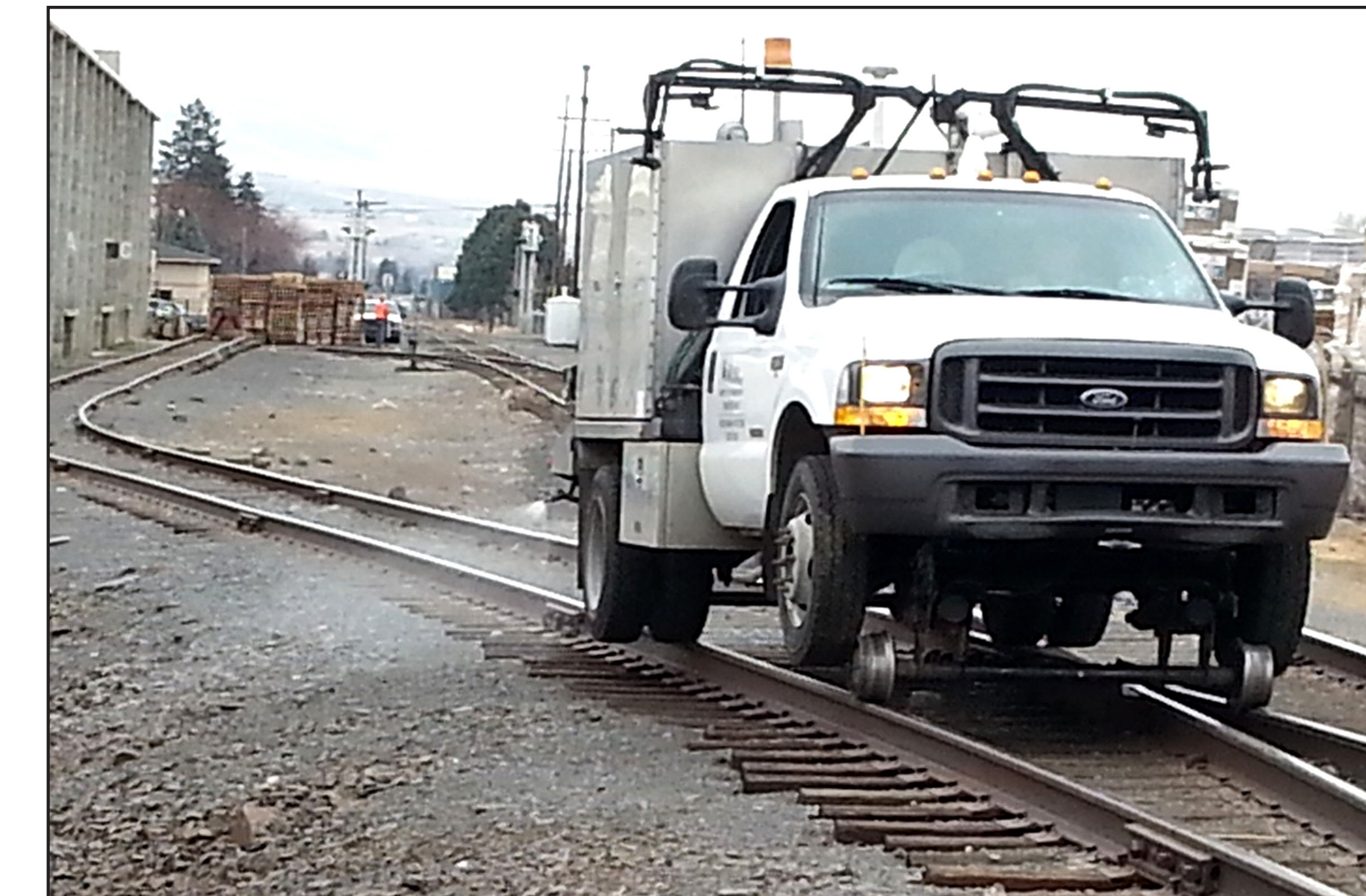
Ferrosafe uses specialized on-track equipment to provide targeted herbicide application for effective vegetation management.
