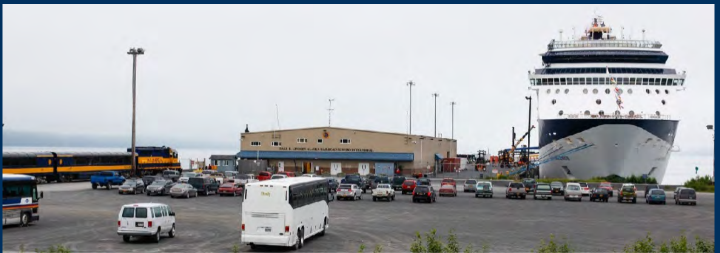
Photo 7-3: Existing Dale R. Lindsey Terminal Building at Seward (Source: Judy Patrick Photography, 2012)
