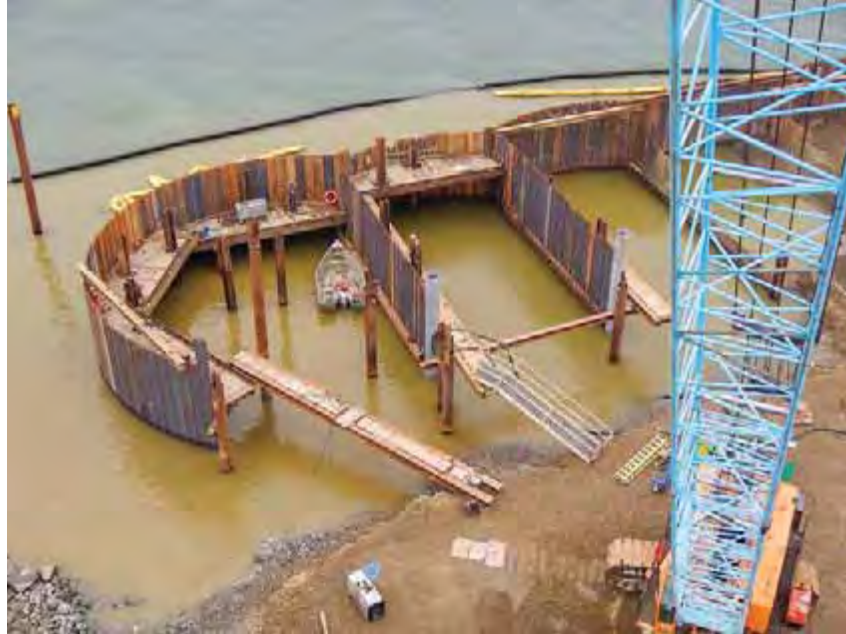
Figure 2 OPEN CELL Templates with Flat Sheet Pile Installed Around the Templates
