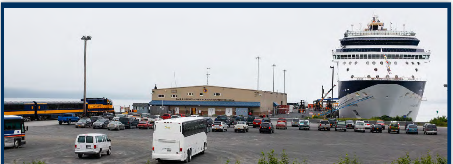
Photo ES-2: Dale R. Lindsey Intermodal Terminal Building at Seward (Source: Judy Patrick Photography, 2012)
