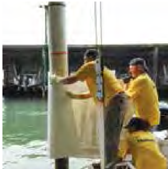
Figure 12 FRP Sheet Being Installed Around a Pile (photo from QuakeWrap, Inc)
