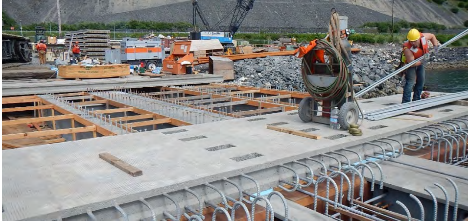
Figure 9 Precast Concrete Deck Panel Set in Place
