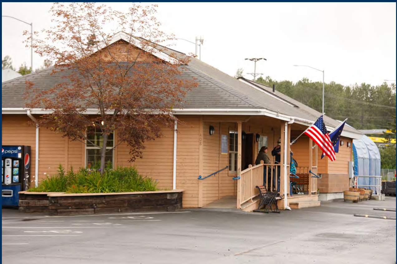
Photo 7-1: Existing Depot Building at Seward (Source - Judy Patrick Photography, 2012)
