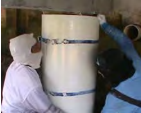
Figure 13 FRP Sheet Wrapped Around a Pile with Straps (photo from QuakeWrap, Inc)
