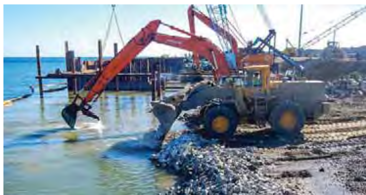
Figure 1 Construction of Crane Pad for OPEN CELL Installation
