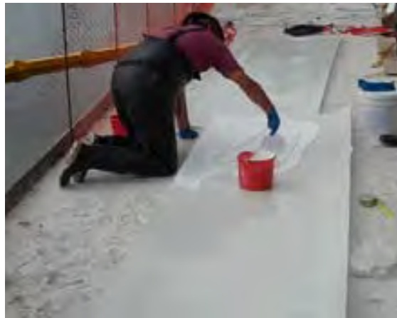
Figure 11 Epoxy Being Troweled onto FRP Sheet (photo from QuakeWrap, Inc)
