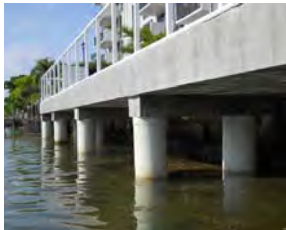
Figure 15 Finished FRP Wrap on Offshore Piles (photos from QuakeWrap, Inc)
