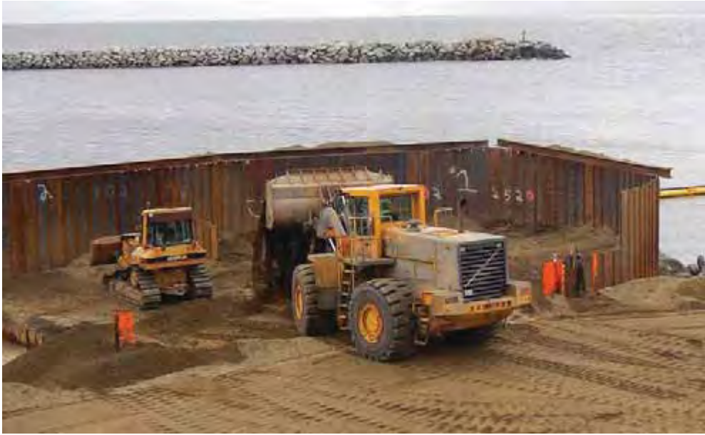
Figure 4 Gravel Backfilling of OPEN CELLS with Standard Earthwork Equipment
