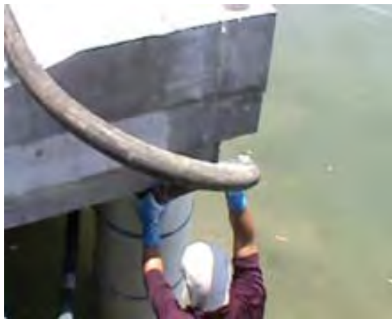
Figure 14 Pumping Grout into FRP Wrap (photo from QuakeWrap, Inc)
