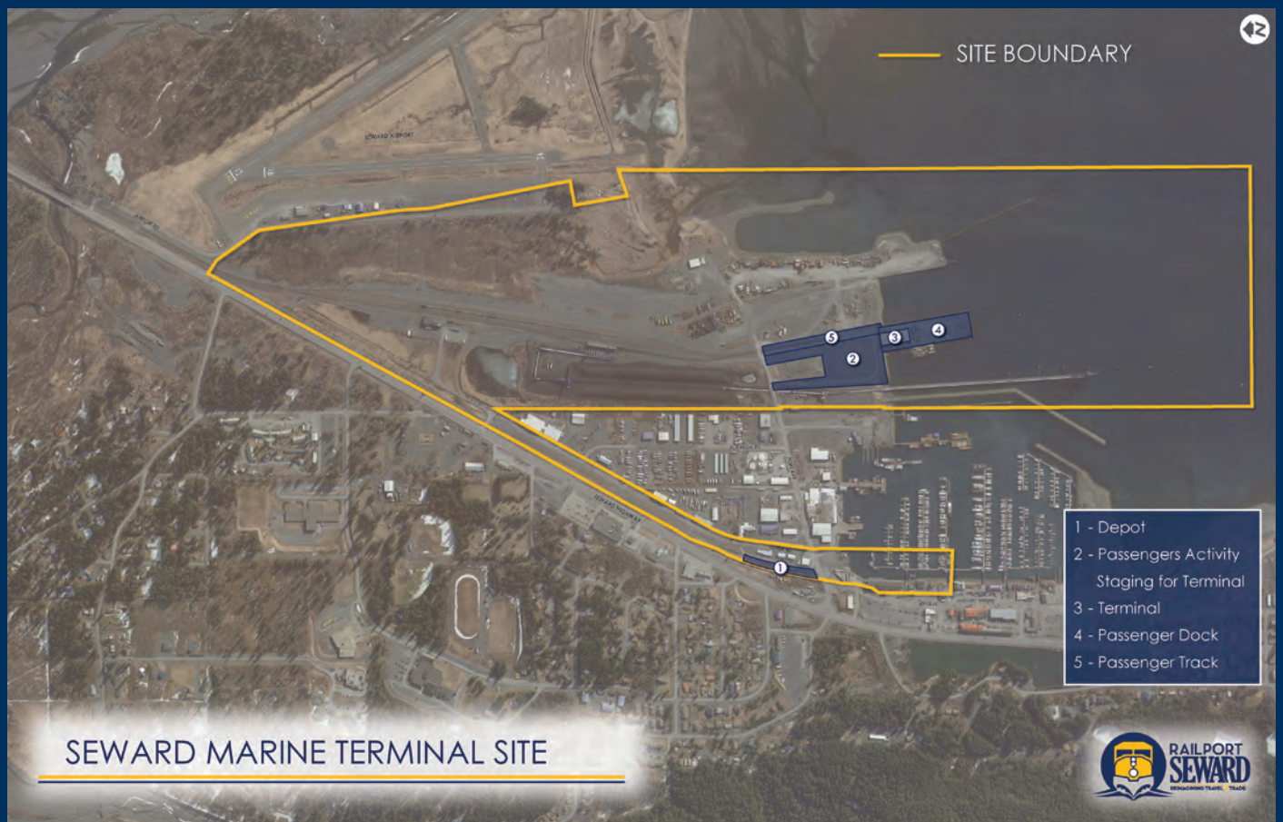
Figure ES-1: Seward Marine Terminal Site and Passenger Facilities
