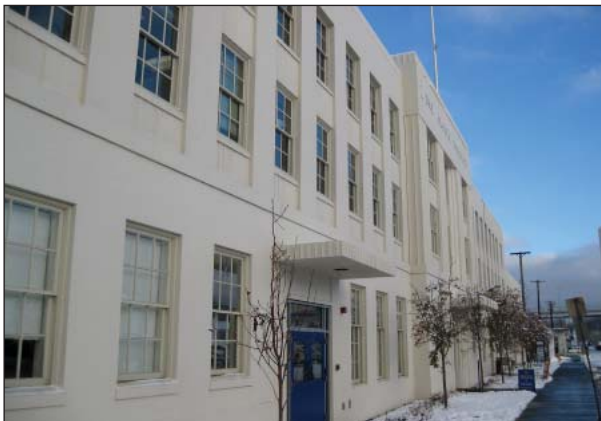
Phase 2a work gives the depot a fresh look with new paint, windows, doors and flag pole.
