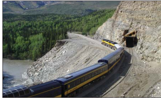
2005: Track is realigned to bypass Garner Tunnel, which is no longer used.
