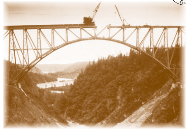
Built in 1921, the 914-foot Hurricane Gulch Bridge at Milepost 284.2 is a remarkable feat of engineering. It is eligible for the National Register of Historical Places. This photo of this iconic bridge is part of the Alaska Railroad's collection of historic photos archived at the Anchorage Museum of History and Art.
