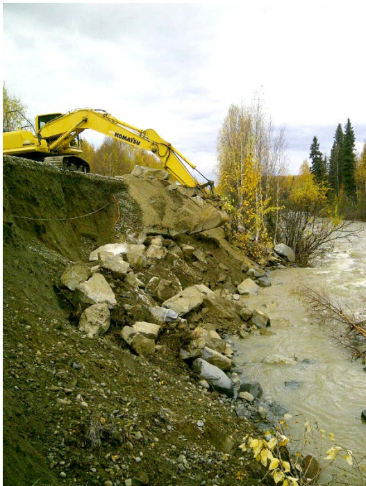
Crews place rip-rap at Sheep Creek to fortify railroad bridge abutment.
