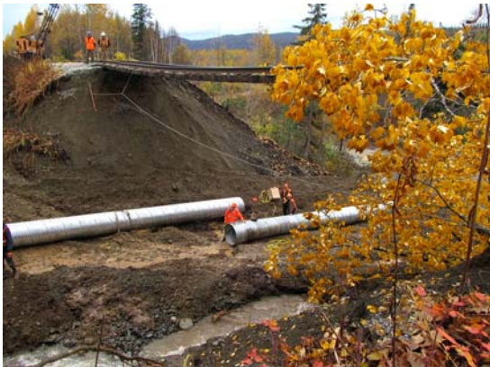
Crews install a culvert under the track at ARRC MP 261 to divert the flood-formed water channel that caused the washout.
