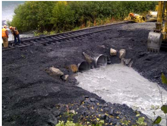
A track washout about 20 miles north of Seward is repaired with newly-installed culverts.
