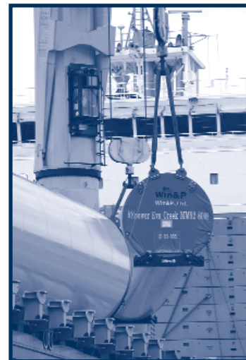
Tower sections unload at the port. (Photo by David Blazejewski)
