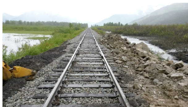
Crews make progress in plugging washout.
