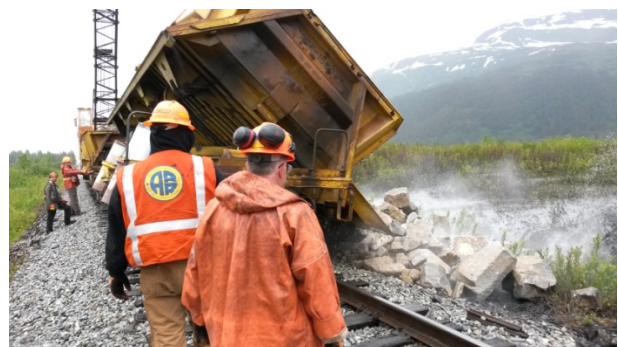
Rip-rap is hauled in by air dump railcars.
