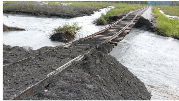
Material is pushed into place to plug the gap,
