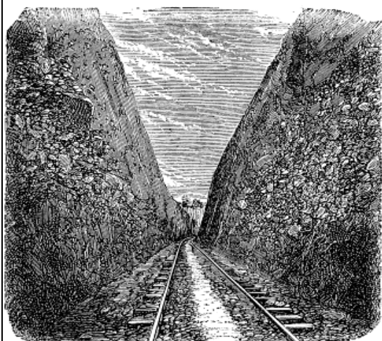
No. III.—BLOOMER CUT, 63 feet deep, 800 feet long.
