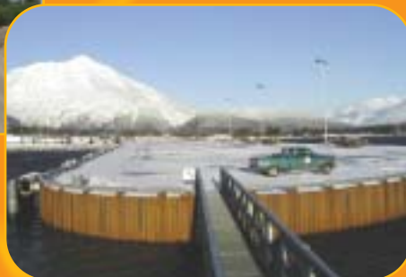
The freight dock in Seward was completed in 2001.
