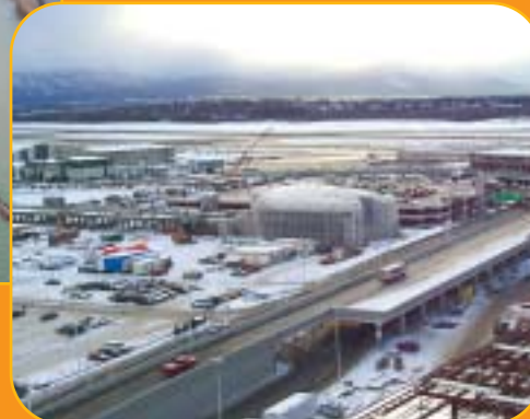
Construction of the Airport Rail Station continued through 2001.
