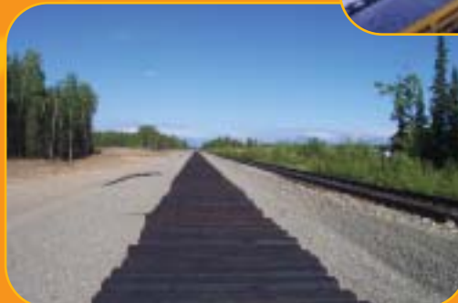
Construction of the new siding at Pittman was completed in 2001.
