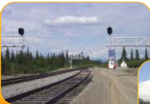
The new Hurricane siding was completed in 2001 and included a powered switch.
