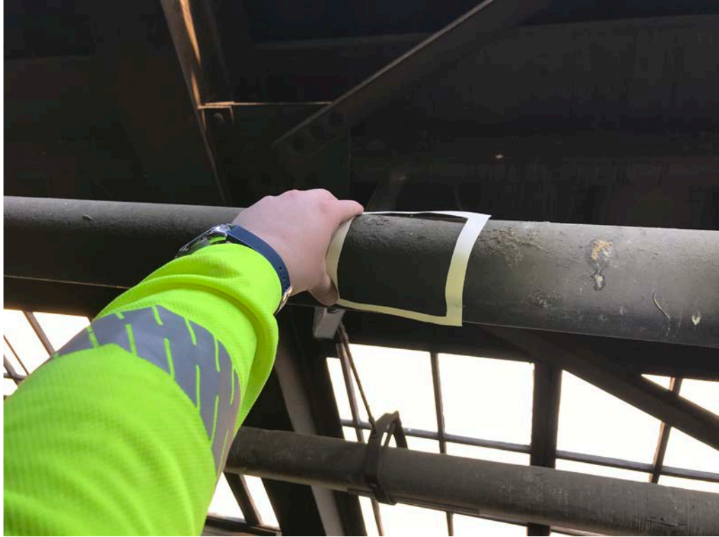
Photo 1: This photo shows the area 18020-Wipe01 was collected. (June 21, 2019)
