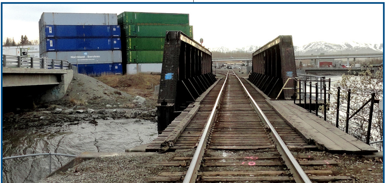
Bridge 114.3 crosses Ship Creek in an industrial area of lower downtown.
