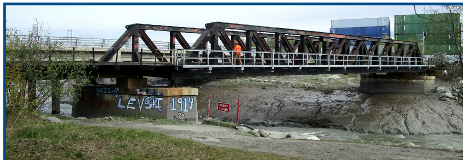
Bridge at Milepost 114.3.
