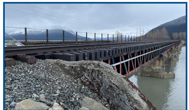
Bridge crosses Twentymile River at MP 64.7.
