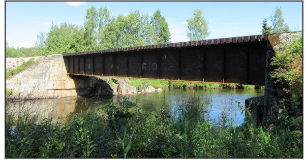
Above: ARRC will replace single-span 80-foot bridge crossing Little Willow Creek at MP 190.5. The project will replace the aging structure with a new 125-foot single-span thru-plate girder bridge.
