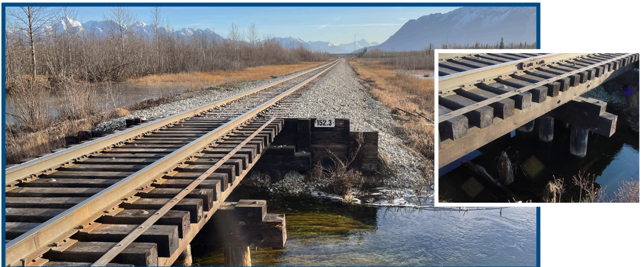
Bridge 152.3 crosses a tributary of Spring Creek south of Wasilla.
