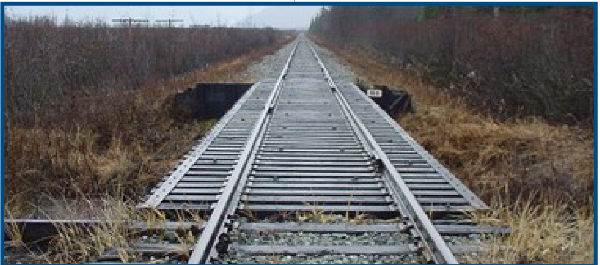
Bridge at MP 56 crosses a tributary of the Placer River.
