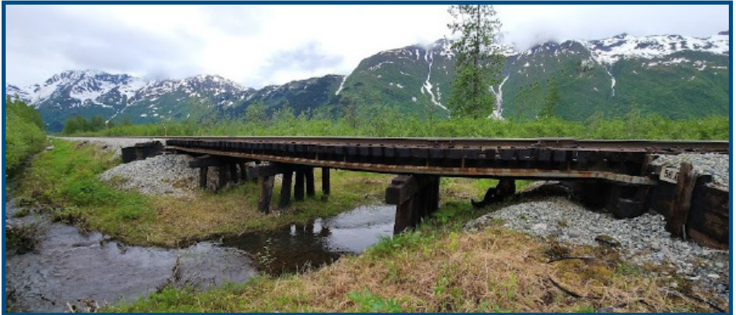
Bridge at MP 56 crosses a tributary of the Placer River.
