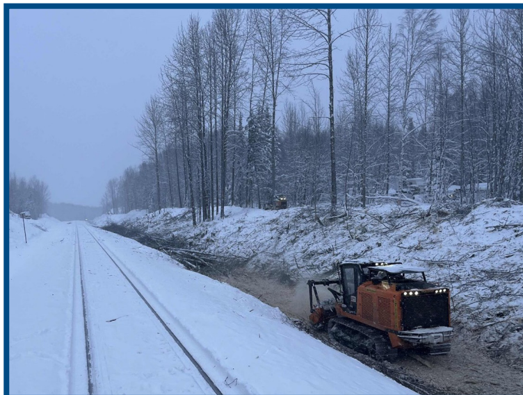
Above: December 2023 vegetation clearing activities in ROW.
