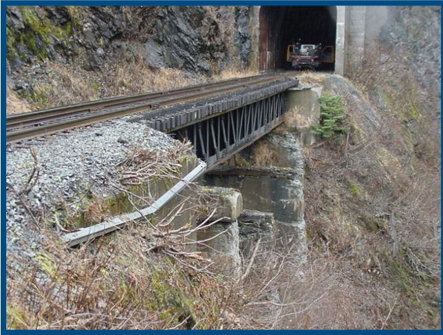
Bridge at MP 52.0.
