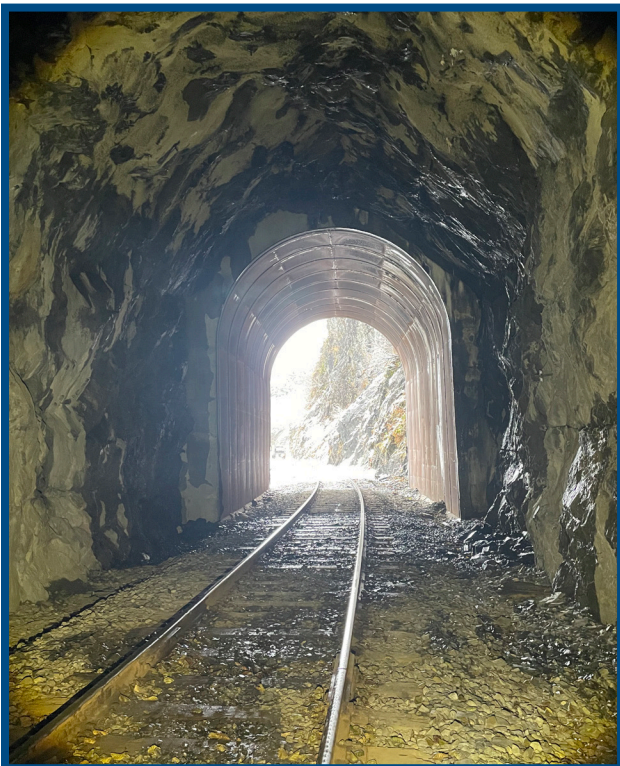
Rock lined interior tunnel.
