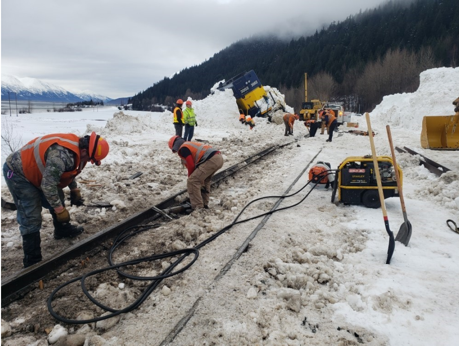
Alaska Railroad crew works to repair the tracks at rail milepost 71.5.
