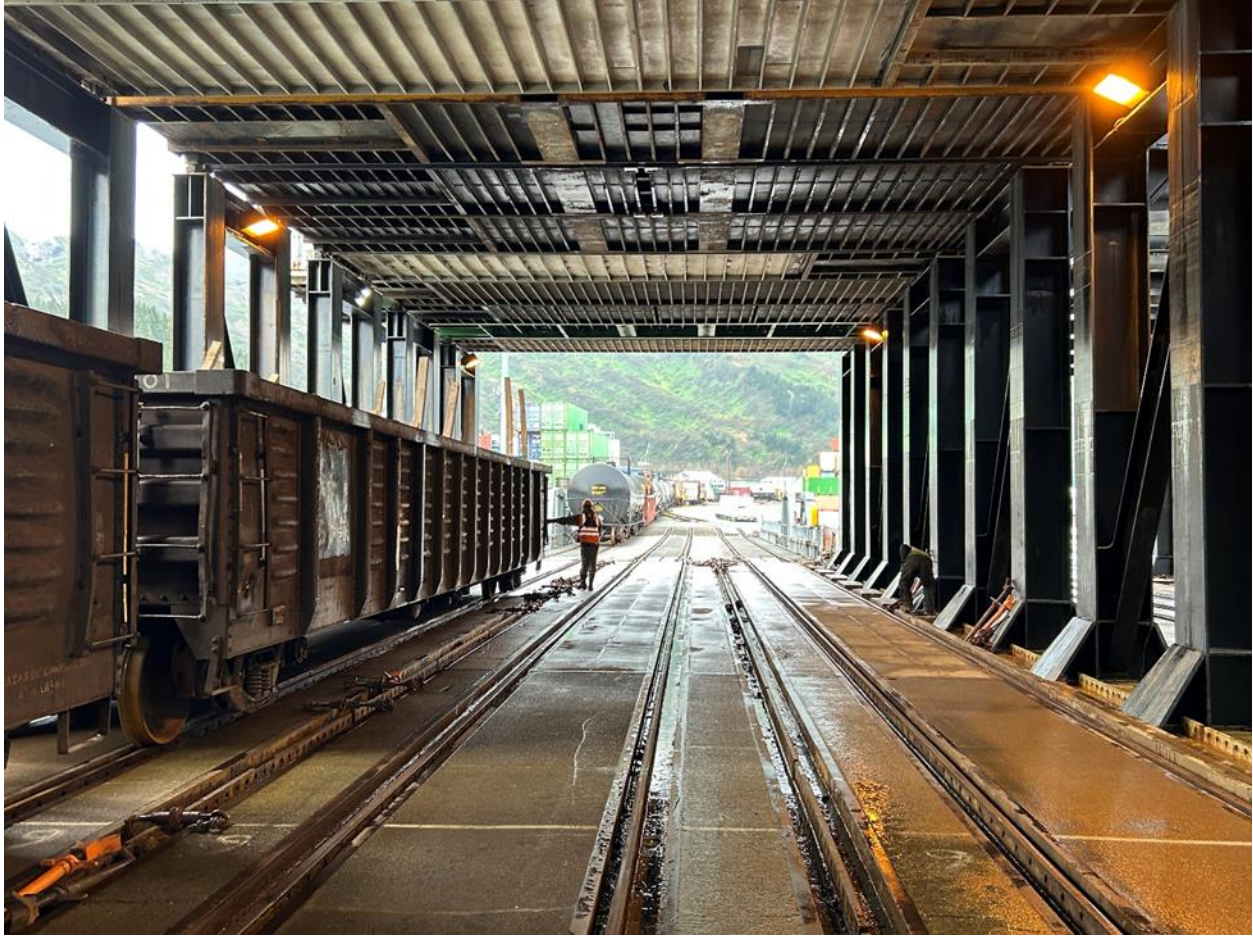
Figure 8. The rail deck on the barge.
