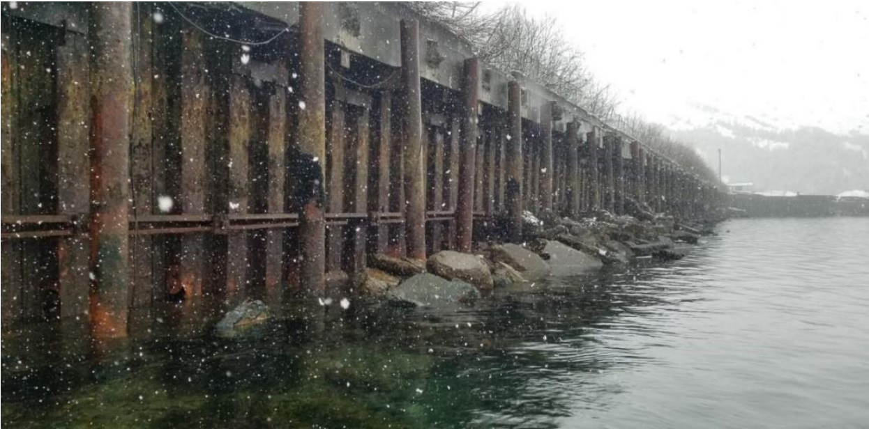
Figure 17. Looking west along marginal wharf bulkhead.
