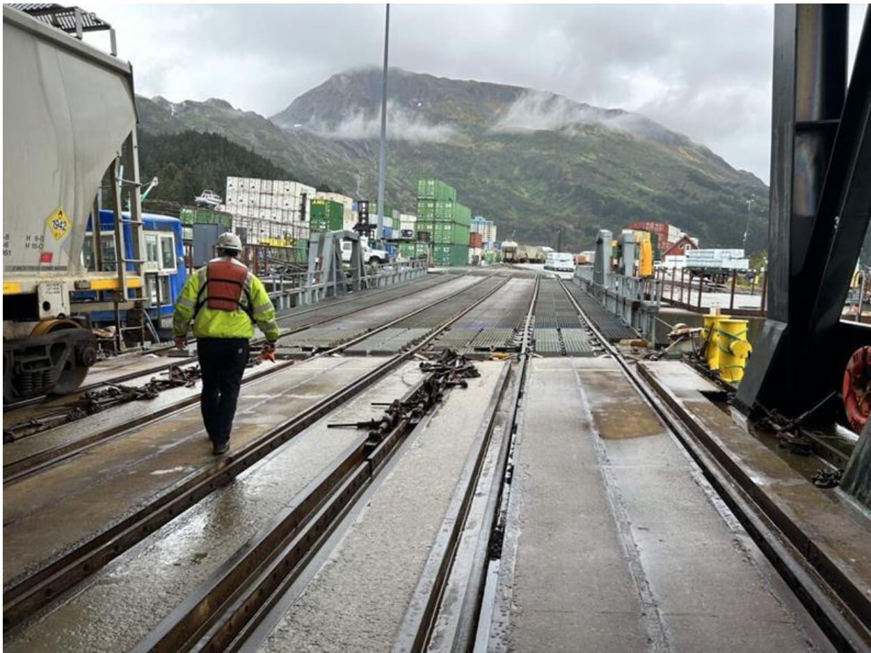
Figure 23. Looking out from barge (west) showing aligned tracks with transfer span tracks.
