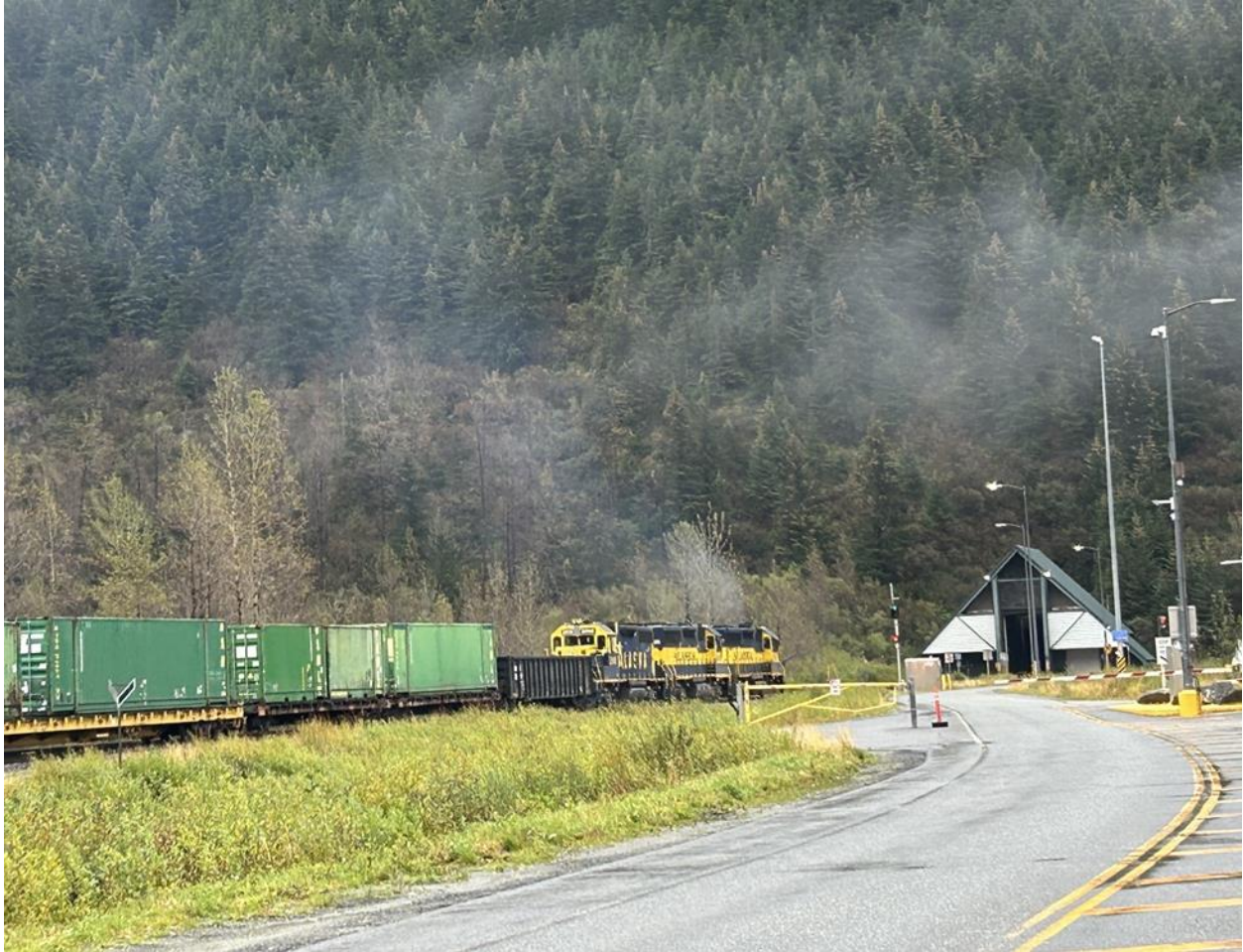
Figure 5. Inbound train preparing to enter the Anton Anderson Memorial Tunnel.
