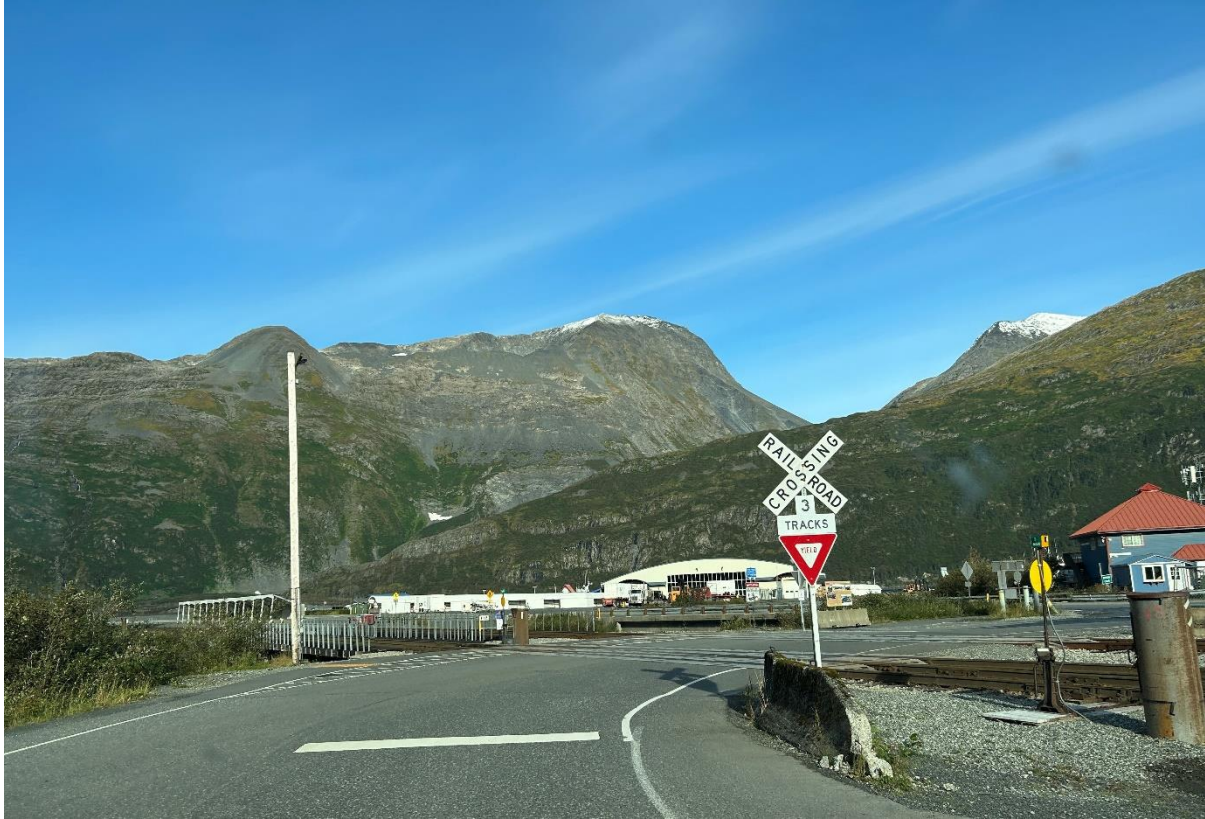
Figure 15. Whittier Street at-grade crossing conflict point.
