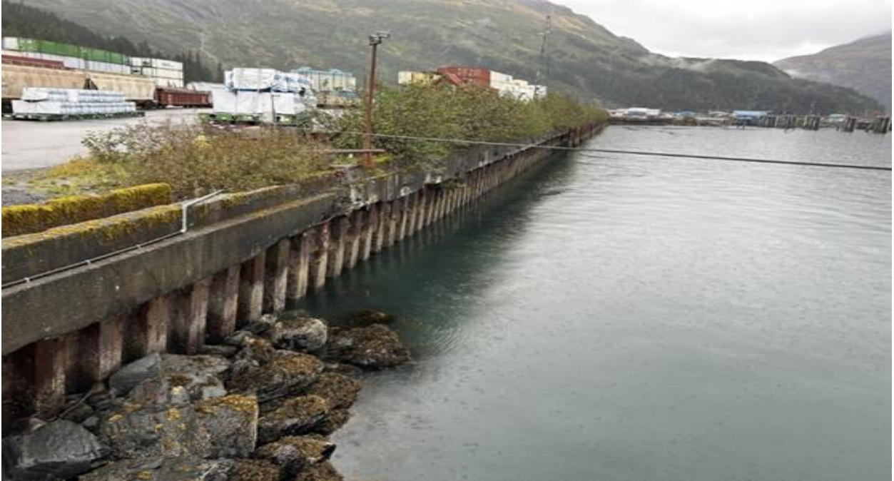
Figure 18. Marginal wharf remnant bulkhead.
