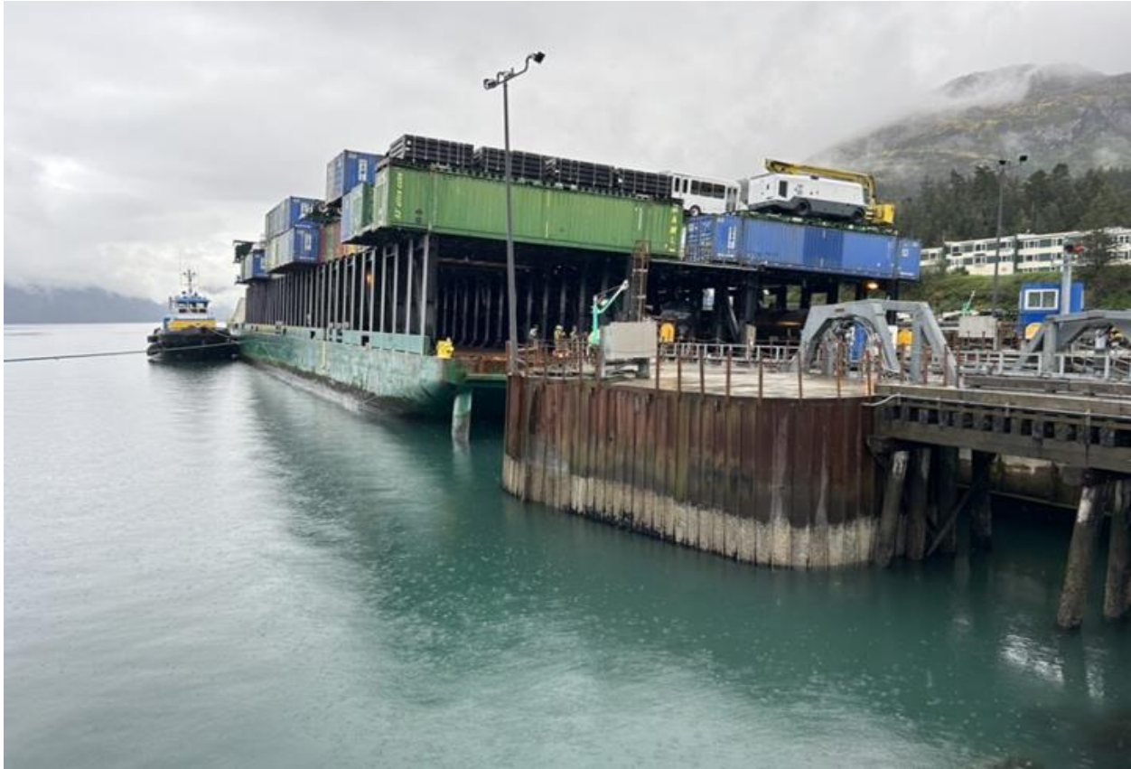
Figure 20. Head end of a barge in barge slip showing berthing structure and loading ramp.
