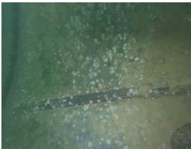
Image 24 – Trestle Steel Pile, typical condition
