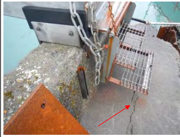
Photograph No. D4-7
