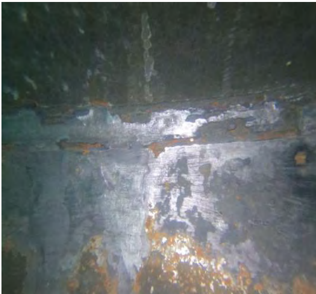
Image 1: Heavy Corrosion
