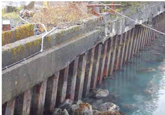
Figure 3 - Marginal Wharf Bulkhead Wall
