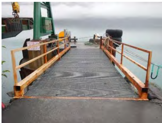
Photograph No. WC-7
