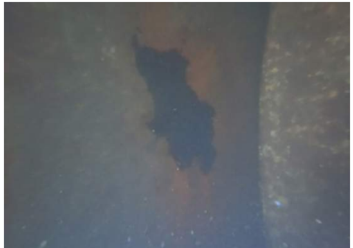
Image 17 – 12"x3' Hole South Side Cell
