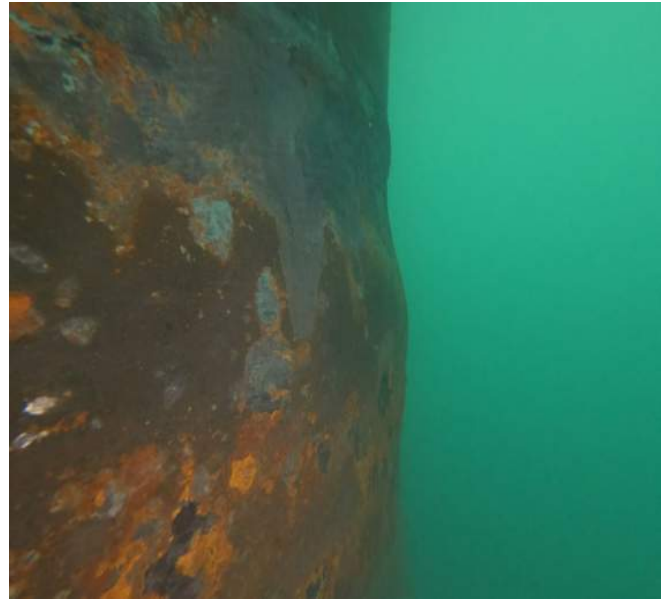
Image 2: Bulbous Deformation
