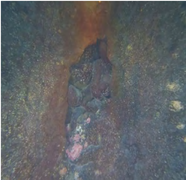
Image 6 - 10"x5" Hole, West Side Cell
