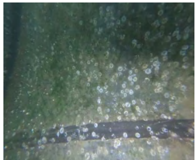
Image 25 – Trestle Steel Pile, Typical Condition
