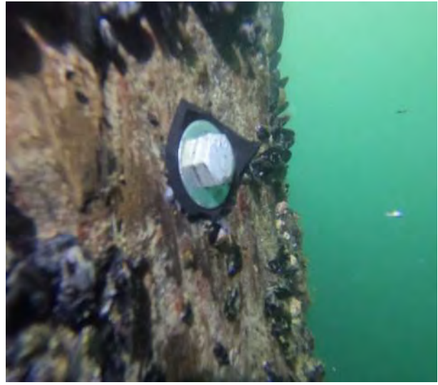
Image 29 – Galvanized Lag and rubber seal
