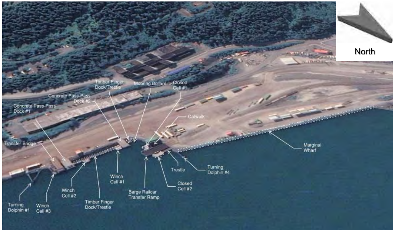
Figure 1 Satellite View of Inspected Components, Courtesy Google Earth
