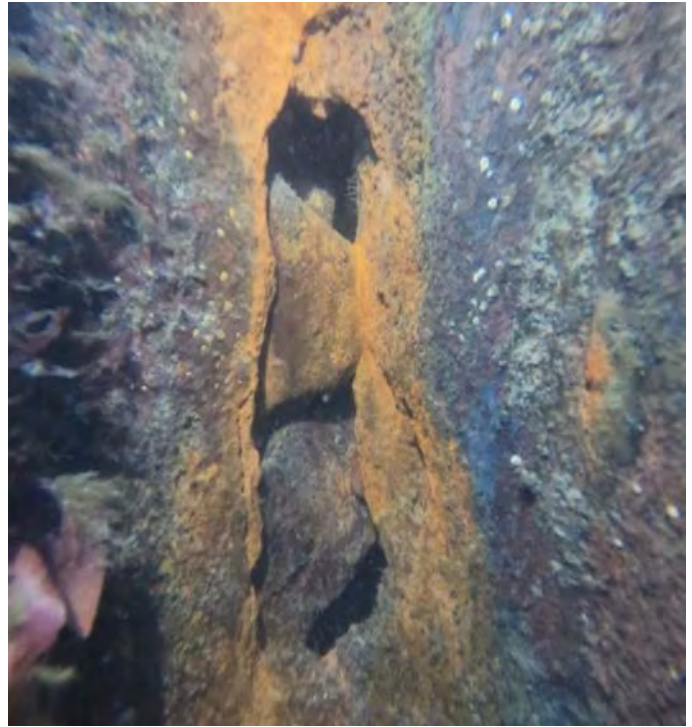
Image 19 – 4" x 11" Hole, South side cell
