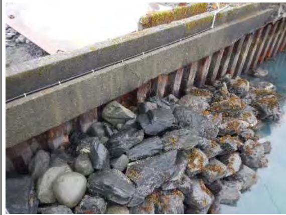
Photograph No. MW-7
