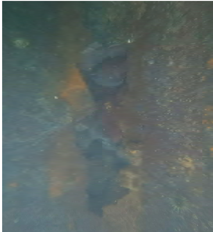
Image 3 - 4" x 18" Hole North Side of Cell
