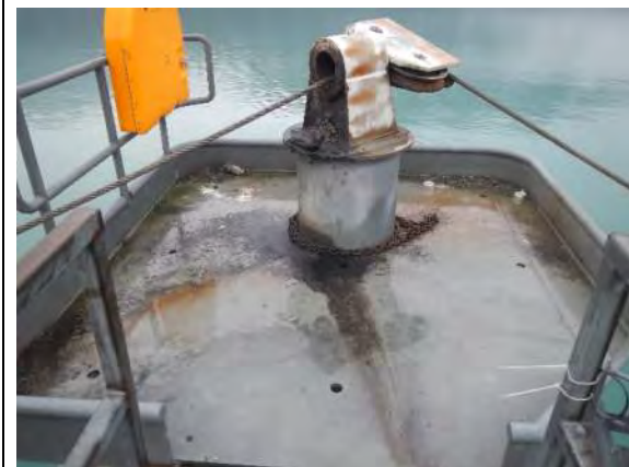
Photograph No. D4-2
