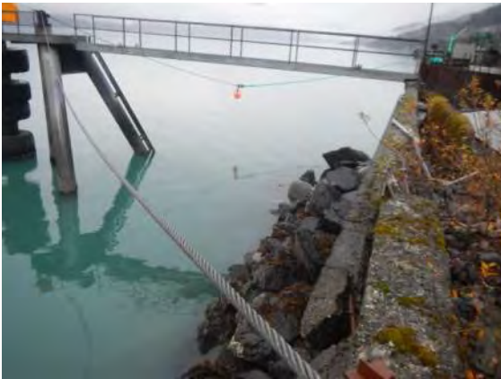
Photograph No. D4-5
