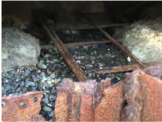
Photograph No. WC-5
