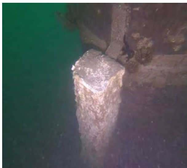
Image 23 – Close up of anode end
