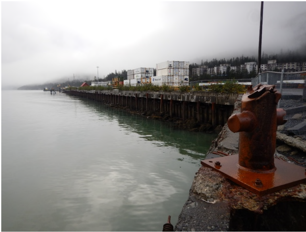
Photo 1: Former Marginal Wharf Location
