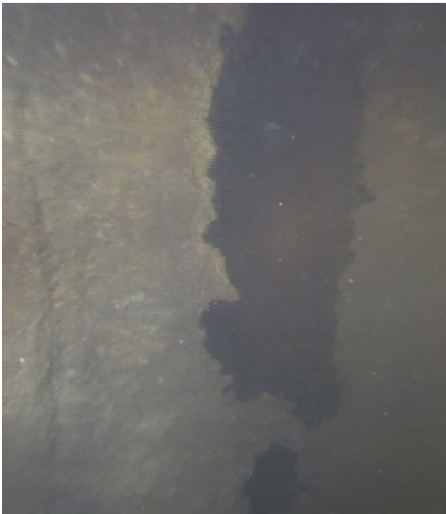
Image 18 – 8" x 5' Hole, South side cell
