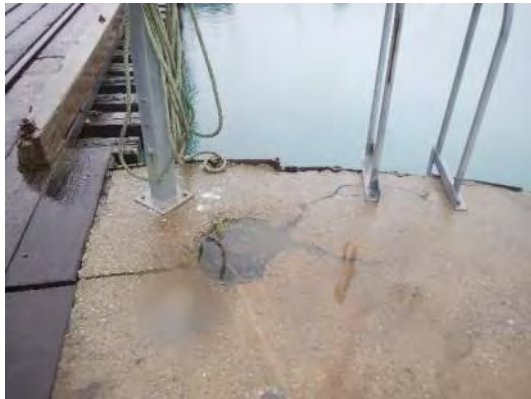
Photograph No. WC-6
