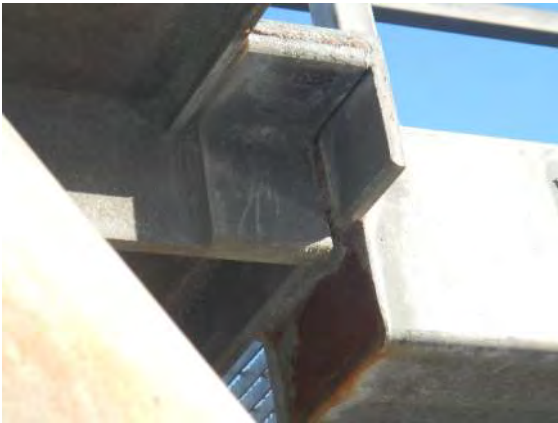
Photograph No. D4-6
