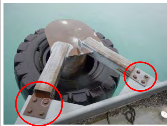
Photograph No. D4-3
