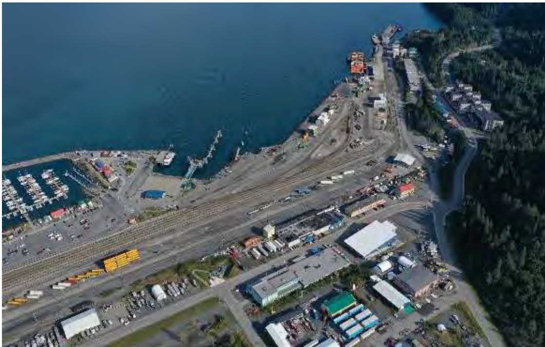
Photo 11: Rail Yard and Dock Area
