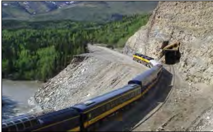
Figure 5-8 Track Realignment near Healy
