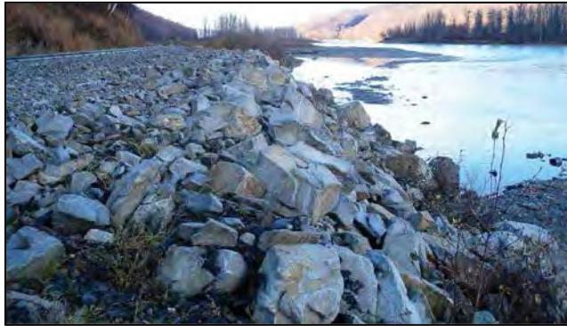
Figure 4-2 Bank Stabilization along the Susitna River
