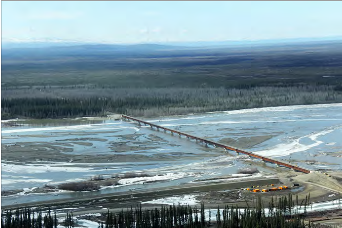
Figure 5-7 Phase 1 - Bridge over the Tanana River
