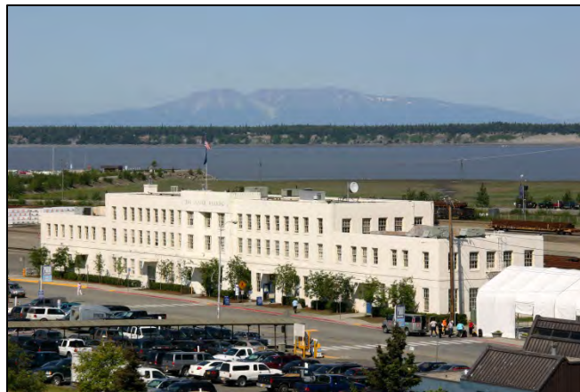
Figure 3-2 Anchorage Railroad Depot
