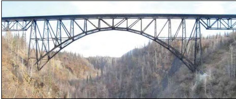
Figure 4-4 Hurricane Gulch Bridge
