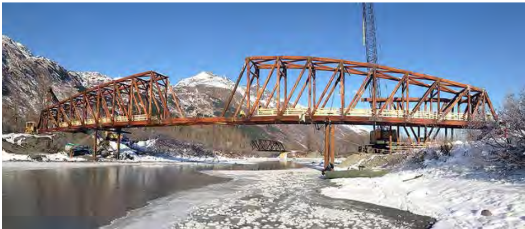
Figure 4-6 Placer River Trail Bridge Under Construction
