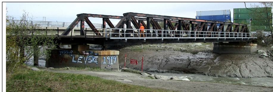
View of bridge at Milepost 114.3.
