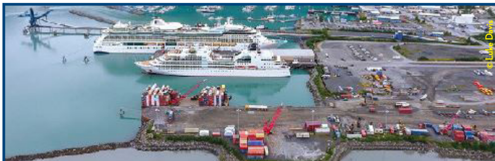
The Freight Dock with Passenger Dock in the background.
