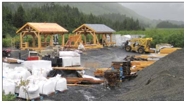
Construction gets underway on the Grandview Whistle Stop site in summer 2011.
