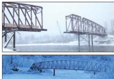
The first of two pedestrian bridges is constructed over Placer River.
