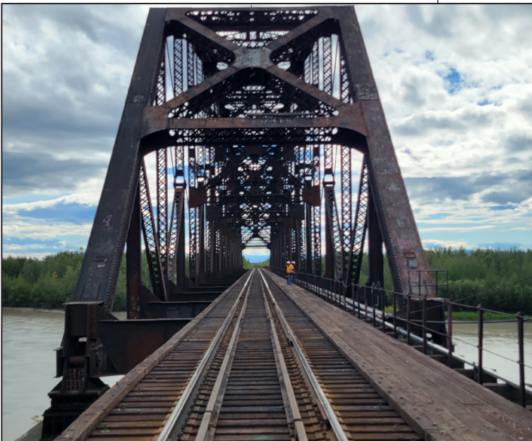
Bridge 413.7 crosses the Tanana River near Nenana.
