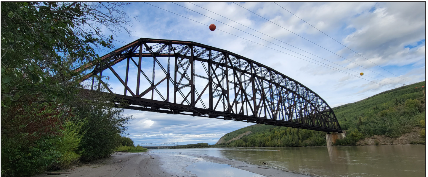
East view of bridge 413.7, the bridge's top chord will be rehabilitated, as well as hangers and interior floor beams.
