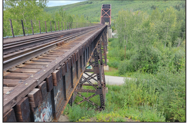
Deck plate girders will be rehabilitated on Bridge 413.7.
