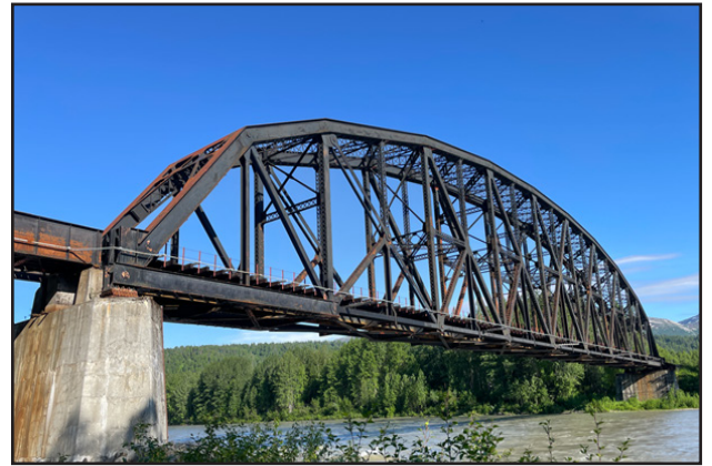
Girder spans will be rehabilitated on bridge 264.1.
