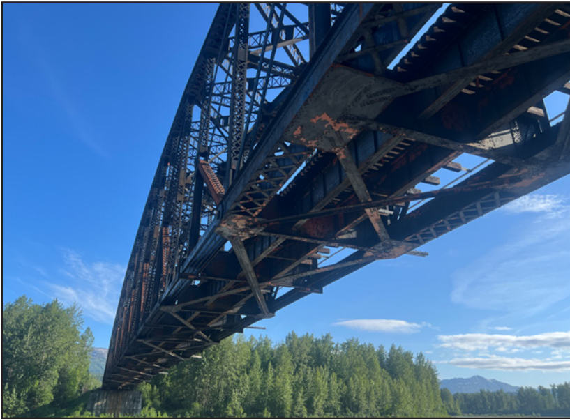
Underside of bridge 264.1 showing lateral bracing used in its construction.
