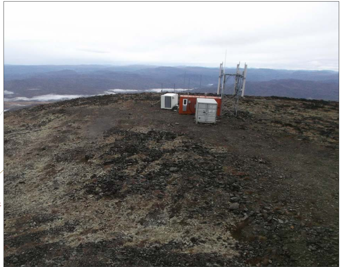
Photograph of site. Looking north.
